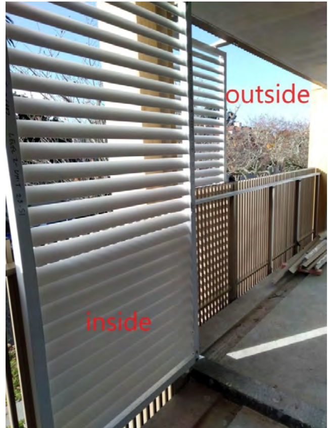
Figure 7: Privacy screens located on the inside and the outside of a balcony
